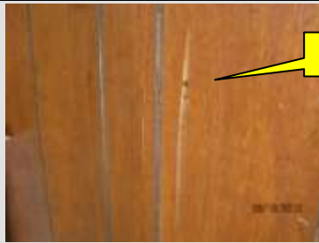
Delaminated siding
